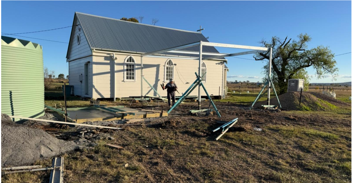
Work for the new Toilet block at Freestone is finally underway.
